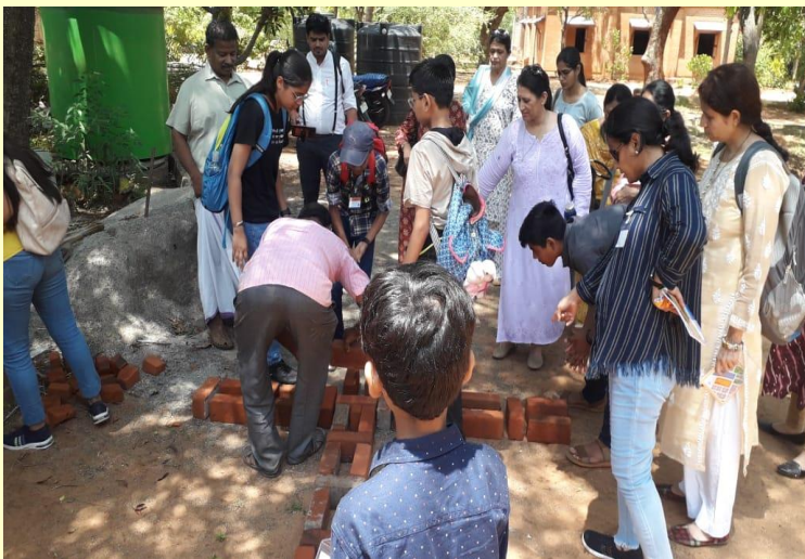
Hands on training - Rat trap model wall construction
