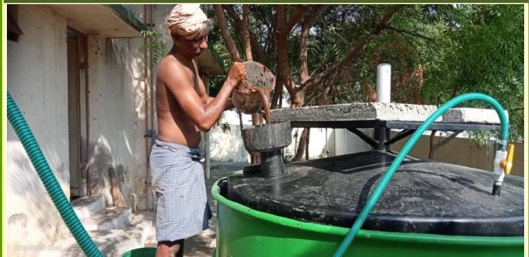
Initially pouring cow dung slurry in the plant for developing bacterial colonies
