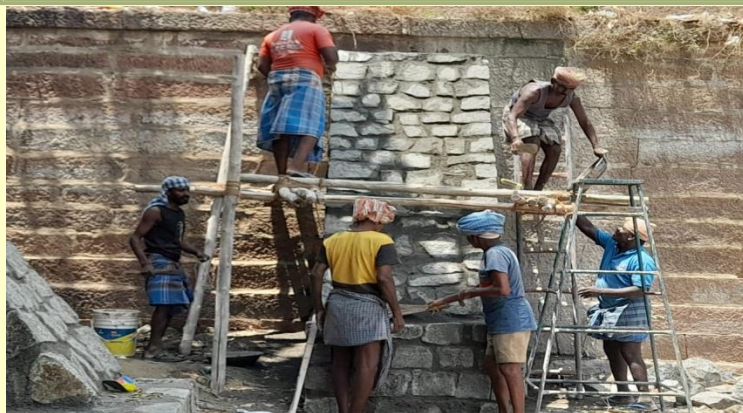
Pier construction is on ...
