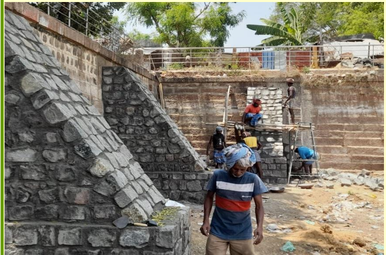
Completed pier supporting the wall
