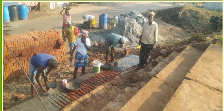
Construction of steps for entry to the Koneri Teertham
