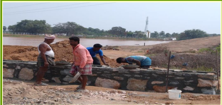
Compound wall work is on ....
