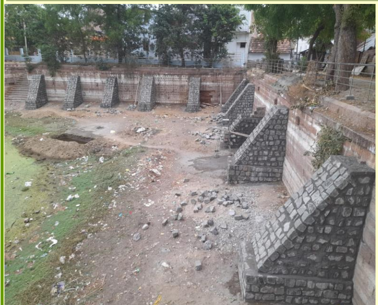
Piers at regular interval to avoid future damage
