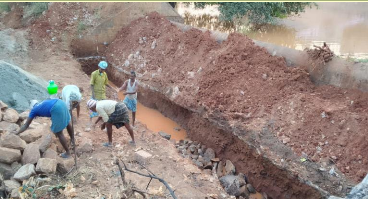
Proper foundation for the compound wall
