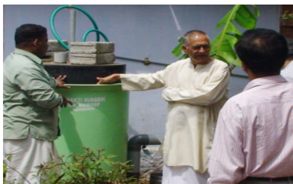
Commissioning the Bio-Methanation plant
