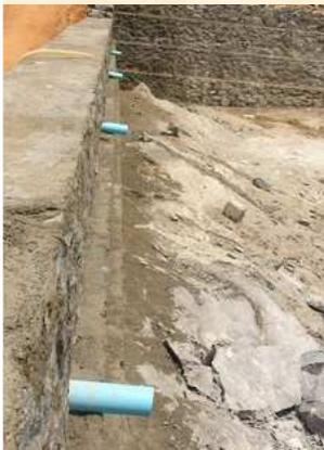
The rain water around the hillock was channelised to the tank and for that channels were made and also structures, in the form of 4' PVC pipes (left) have been embedded in the walls of temple tank. Deepened, ready with proper infrastructure constructed and aligned topographically to receive rain water, now the structure started expecting the monsoons to fill it with water and transform the landscape with the precious resource for life.
