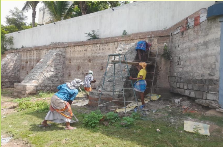
Construction of piers is on ... to strengthen the wall
