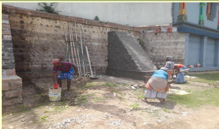
Curing work is on ....
