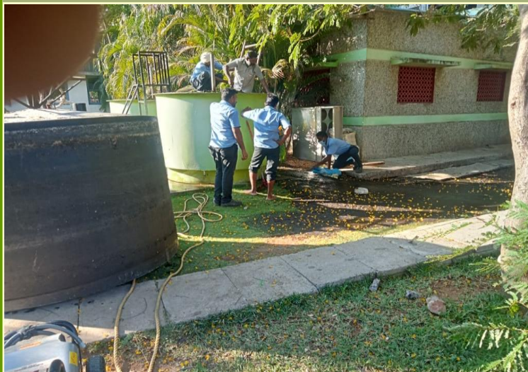
Cleaning of the digester is on ...
