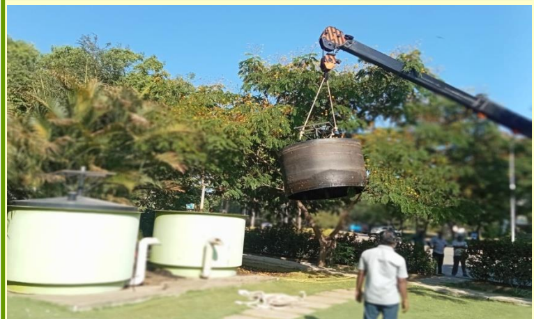
Placing of gas holder above the digester through Crane
