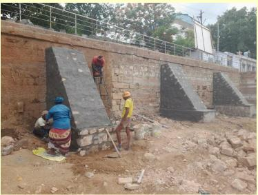
Touch up work and curing by water the Piers constructed for supporting the wall
