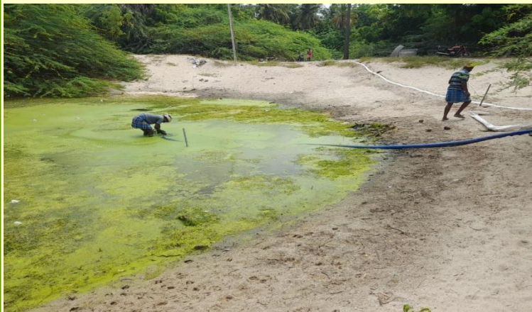
Pumping out the stagnant water and preparing for proper desilting
