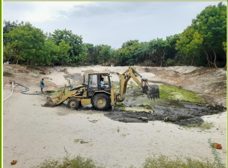
Desilting and deepening the area for constructing the Teertham
