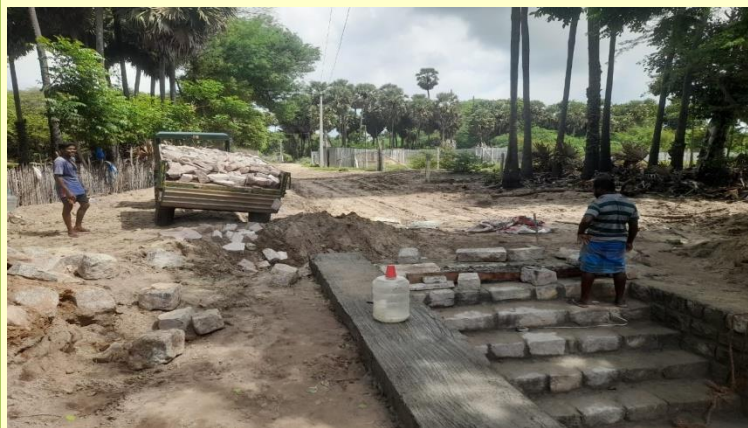
Steps construction for the entry of the Teertham
