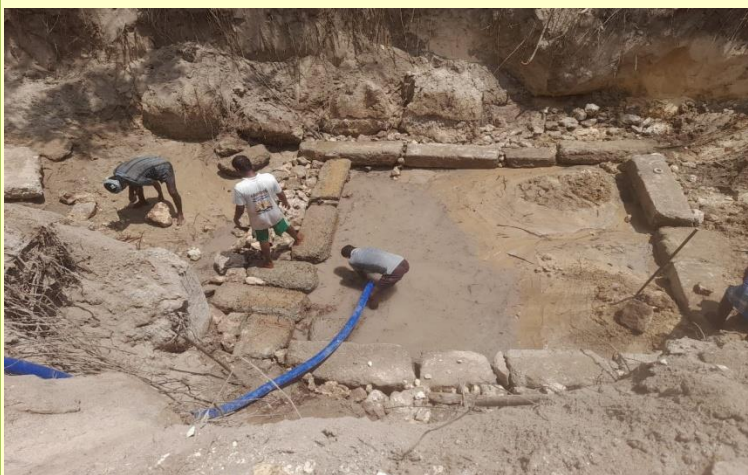
Dewatering the area for proper construction of foundation
