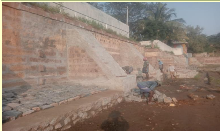
Downloading the stones for constructing a wall
