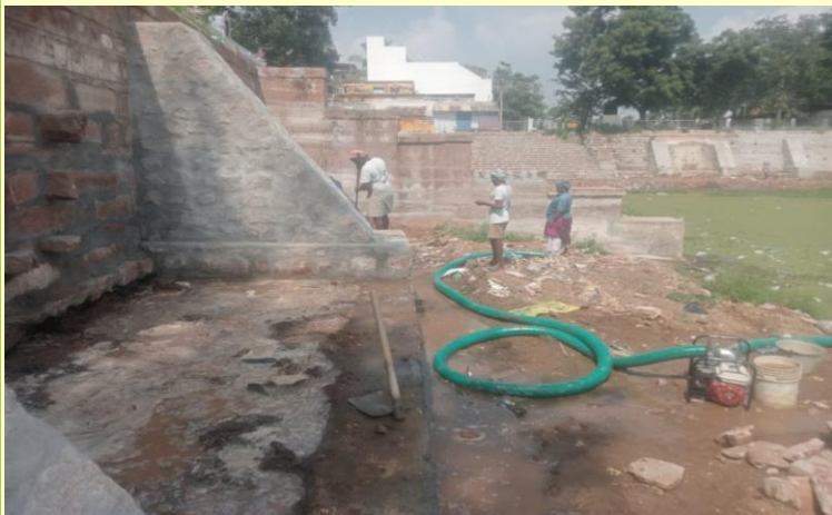
Workers preparing themselves for starting the work
