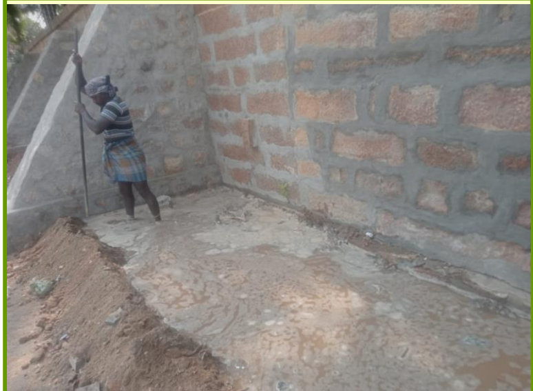
Digging work is on ...
