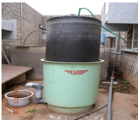
**Figure 1:** Biogas production using mushroom spawn waste
